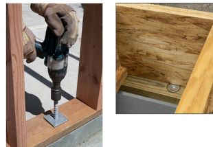
Post installed anchors = Screw Anchors
